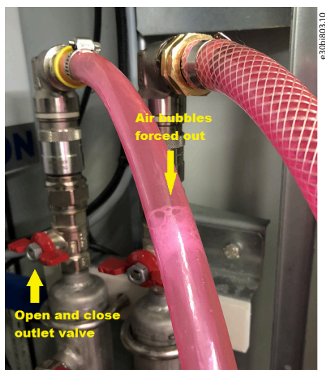
Illustration 75: Removing the Air
