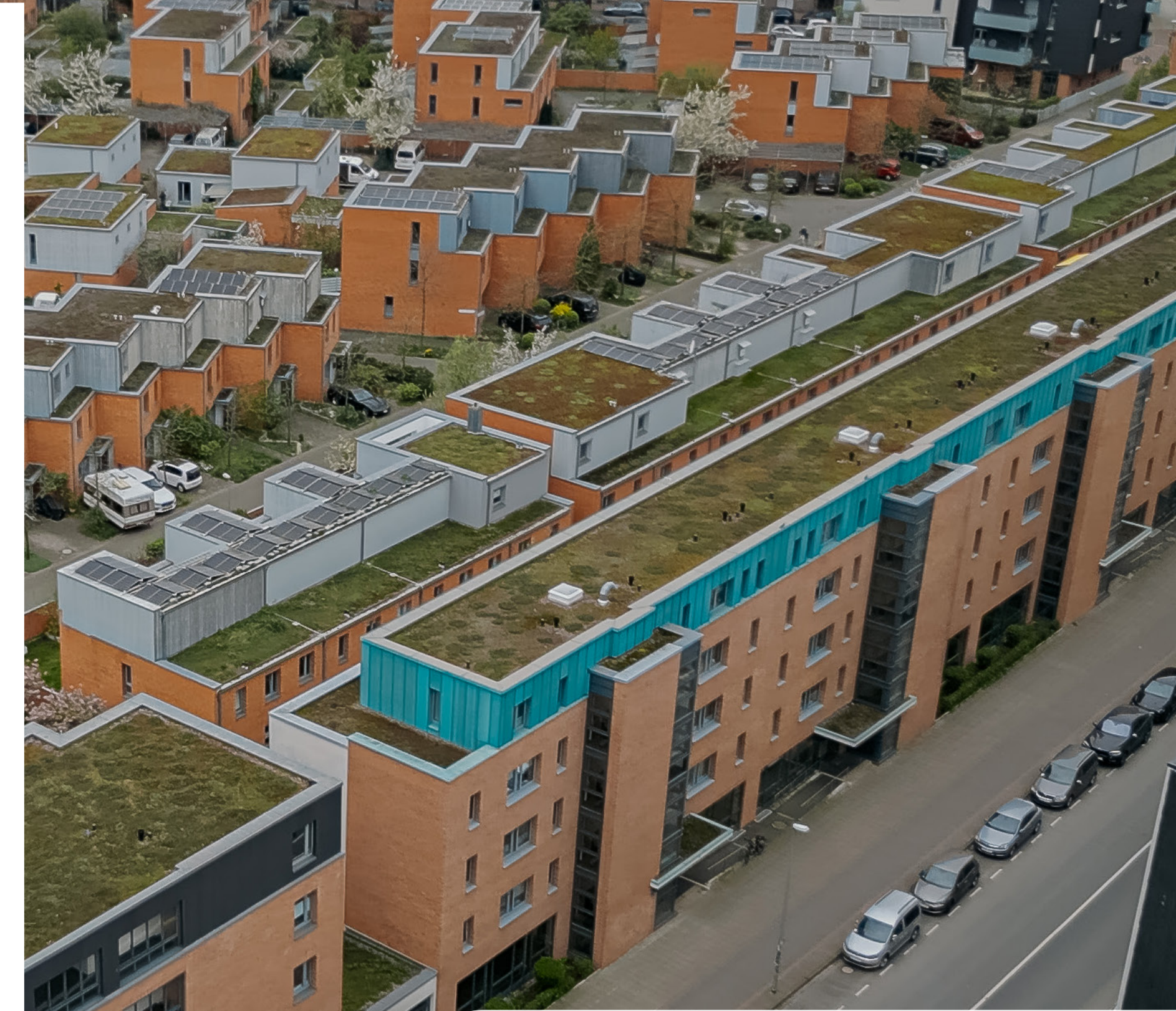
Fig. 7-9: The use of Leanheat® Building was tested as part of a pilot project conducted in a total of 24 properties, including properties of the housing association Ostland (right). For this, enercity equipped the buildings' substations with, among other things, network-enabled Danfoss ECL 296 district heating controllers (bottom left). Image source: Danfoss
