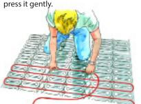
2. Clip plates together. Cut plates with jigsaw if necessary.
