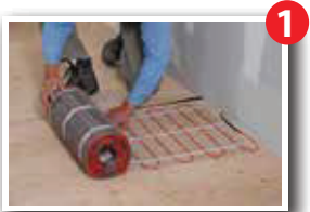
Unroll the self-adhesive mat onto the floor
