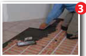
Install tile / floor coverings
