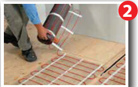
Cut the mesh to turn Never Cut the RED Cable
