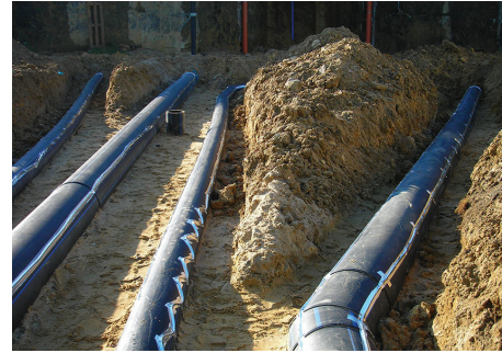
Pipeline in Strzelce Opolskie, Poland
