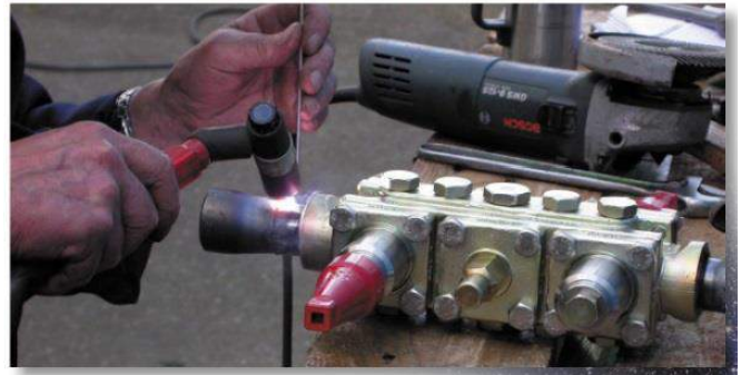
Direct welding without disassembly
