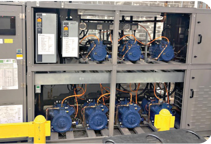
← Figure 3 shows the rack retrofitted with three Danfoss BOCK compressors in the low-temperature (LT) suction group (above) and four in the medium-temperature (MT) group installed with proper bracing. The variable frequency drive (left) sets the specific frequencies cited in the accompanying charts.
