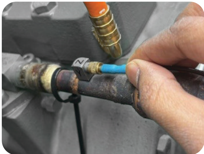
↑ Figure 4 shows the LT1 compressor discharge vibration measurement point (see Chart 1).
