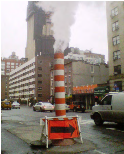
FIGURE 3: A chimney for dispersion of condensation from the steam distribution network. The condensation can be caused by water coming into contact with the steam pipes being boiled or leakage of the steam pipes.
