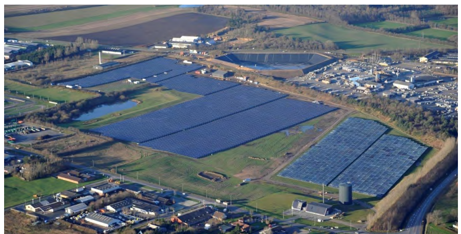
FIGURE 2: Vojens solar heating plant and the storage pit under construction
