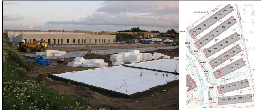
FIGURE 5: Low temperature DH supply for an area in Lystrup/Denmark. Construction site and area plan.
