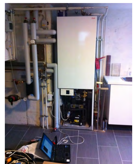
FIGURE 4: y-Booster substation installed in a test house in the Northern Copenhagen area.
