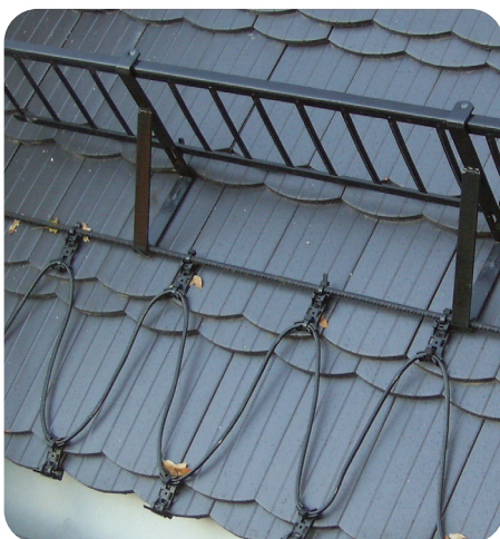
Roof edges and gutter with heating installation.
