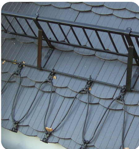
Roof edges and gutter with heating installation.
