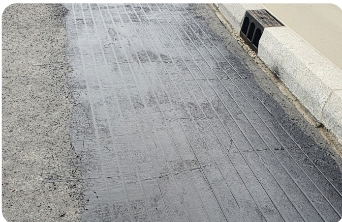
Fig. 1. DEVLasphalt™ heating cable under the first layer of Road asphalt rolled by a hand drum
