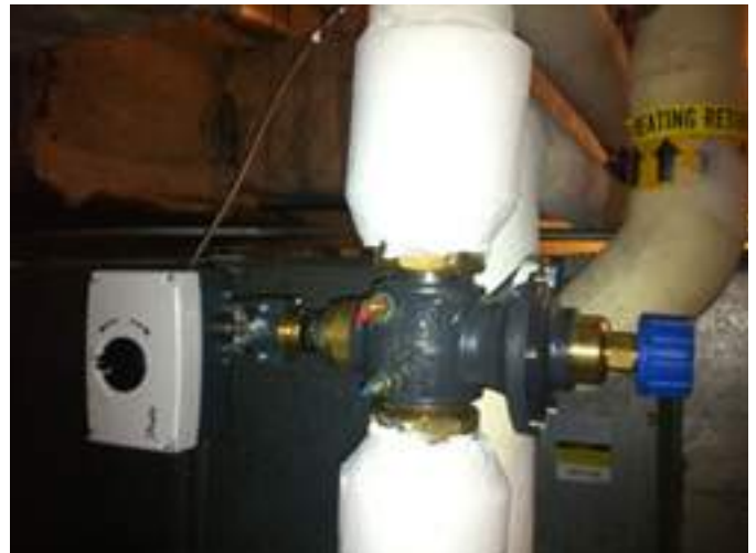
Newly installed Danfoss Pressure Independent Control Valve
