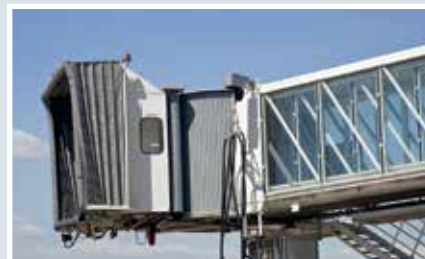
Special air conditioning application (boarding bridges...)
