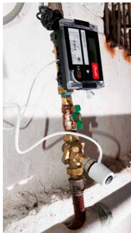
Increased insulation and new windows are not enough to realize the full potential of energy efficiency in buildings with one-pipe heating systems. To get the full benefit from the investment, it is necessary to modernize the one-pipe heating system. Previously, it was generally believed that you had to perform a full-scale conversion to a two-pipe solution. However, Danfoss decided to
