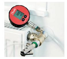
To ensure maximum energy savings the renovated heating system was commissioned with using the dP tool<sup>™</sup>. This simple tool measures the available differential pressure directly in the *Dynamic Valve*<sup>™</sup>. The pump pressure of the Grundfos MAGNA was lowered while the required differential pressure in the furthest located valve stayed intact.
