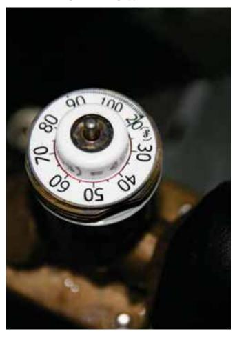
According to Winkler, the AB-QM valve introduced a number of benefits, beginning with ease of installation. The valve eliminates the need to install numerous control elements. As a result, installations of large HVAC systems with AB-QM valves can be accomplished in steps without requiring adjustment to already running parts. And, once a system or part is completed, it is ready for operation. The correct flow can be adjusted in one simple step, without the use of tools.
