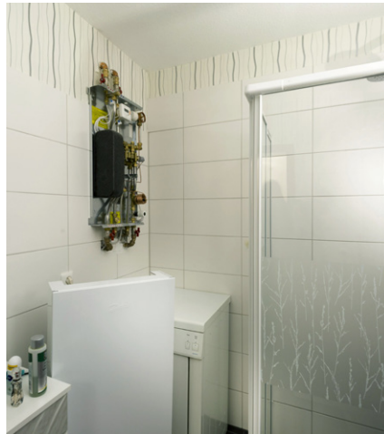
Danfoss' Akva Lux II TDP Reno flat stations can be installed in a compact footprint...
