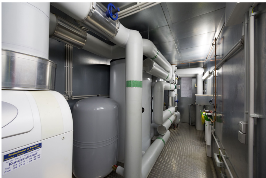
The shipping container on the roof contains the entire heating system – a gas-heated condensing boiler by Brötje with buffer tanks and MSR technology.
