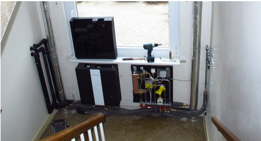
The flat stations are easy to install outside the apartments while residents remain in their homes, as the apartments' kitchens and bathrooms are conveniently located relative to the stairwell.
