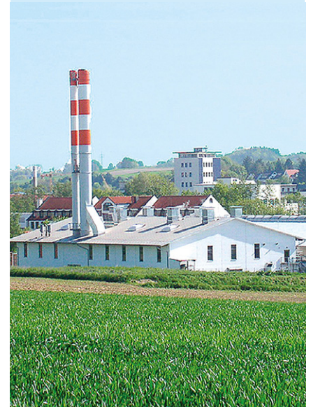
View of the Pfaffenhofen biomass CHP plant - it supplies steam for the baby food manufacturer Hipp and the local hospital. In addition, district heating is supplied to other industrial and commercial enterprises, municipal facilities and more than 100 private consumers.
