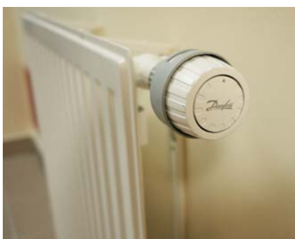
Thermostatic sensor head RA 2920
