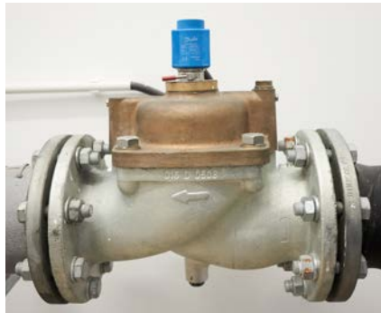
Solenoid valve EV220B
