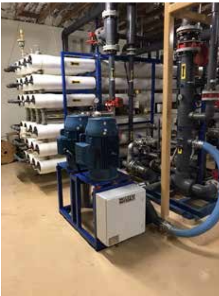
Two APP 26 pumps from Danfoss replacing one centrifugal pump
