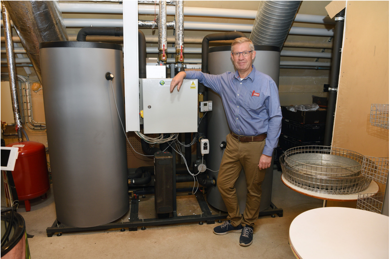
"It just runs by itself," Hans Jørgen Andersen said. The new heat recovery unit from Danfoss heats up 3,400 sqm and also ensures that there is plenty of hot water for the store's butcher and bakery. When there is a baker and a butcher in a supermarket, then there is a high consumption of hot water for cleaning. The excess heat from the refrigeration units handles this as well.
