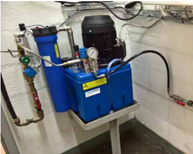
UPW pump unit using a PAH 10 pump
