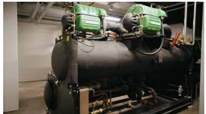
Figure 3: Turboline oil-free chiller by Clint
