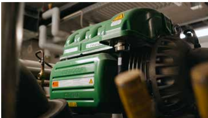
Figure 2: Danfoss Turbocor TG compressor operating with R1234ze
