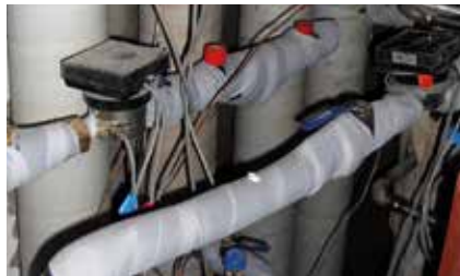
Danfoss ASV balancing valves and energy meters were installed in the technical room for each group of four apartments.
