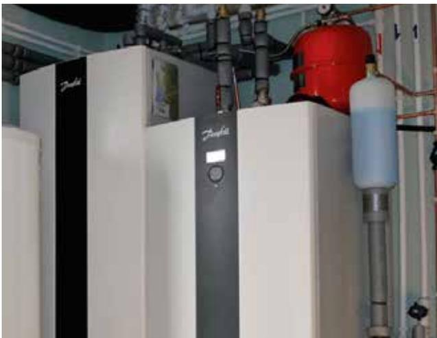
Figure 20 Sample installation of ground source heat pump: DHP-L Opti Pro+ and DWH Opti
