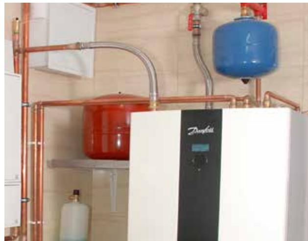
Figure 21 Sample installation of ground source heat pump: DHP-H Opti Pro+
