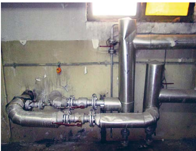
Heating station “Cipelići” before reconstruction
