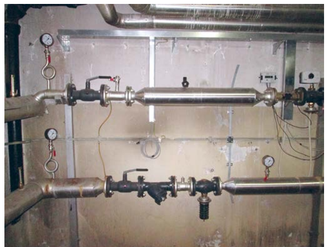
Heating station “Cipelići” after reconstruction
