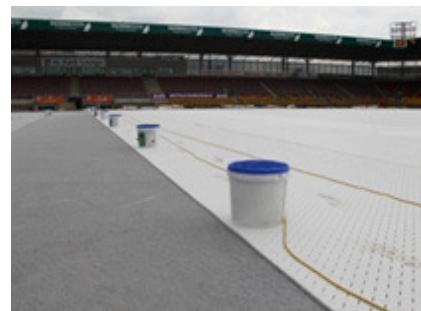
Shock pad, laying out
