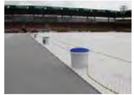
Shock pad, laying out
