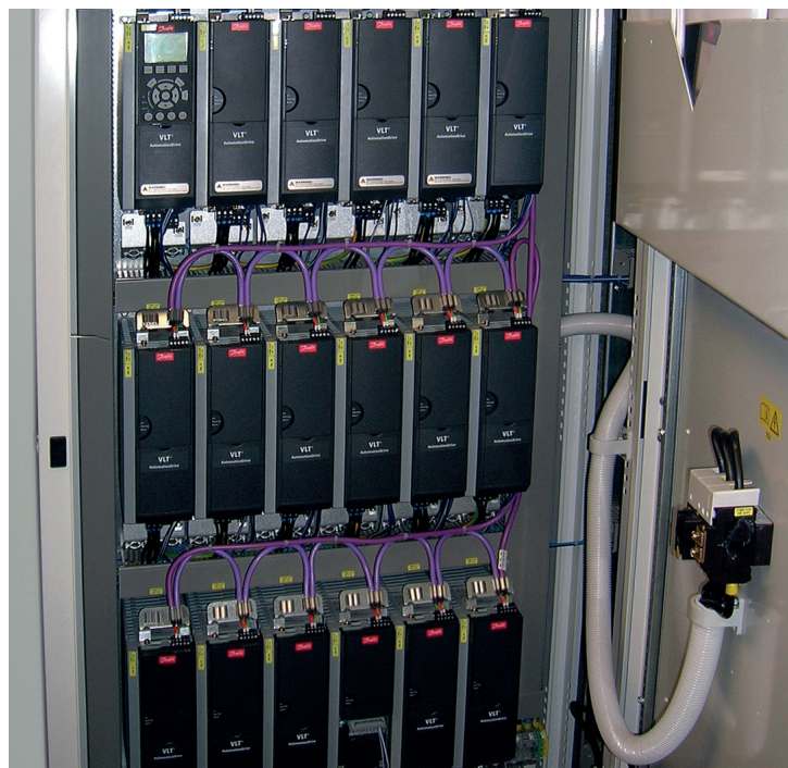
AC drives can be installed centrally in cabinets or decentrally near the drive system. Both concepts have their advantages and disadvantages.
