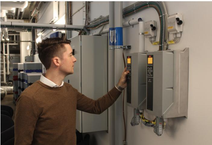
Jacob Haulrich, Nordomatic, continues: "We also use the new VLT® Pressure Transmitter PTU 025 pressure transmitter unit, which monitors air filter clogging and air volume through the ventilation fans. We can obtain the values via BACnet, and because this unit has four pressure transmitters, it has resulted in elimination of three pressure sensors, including cabling, per system".
