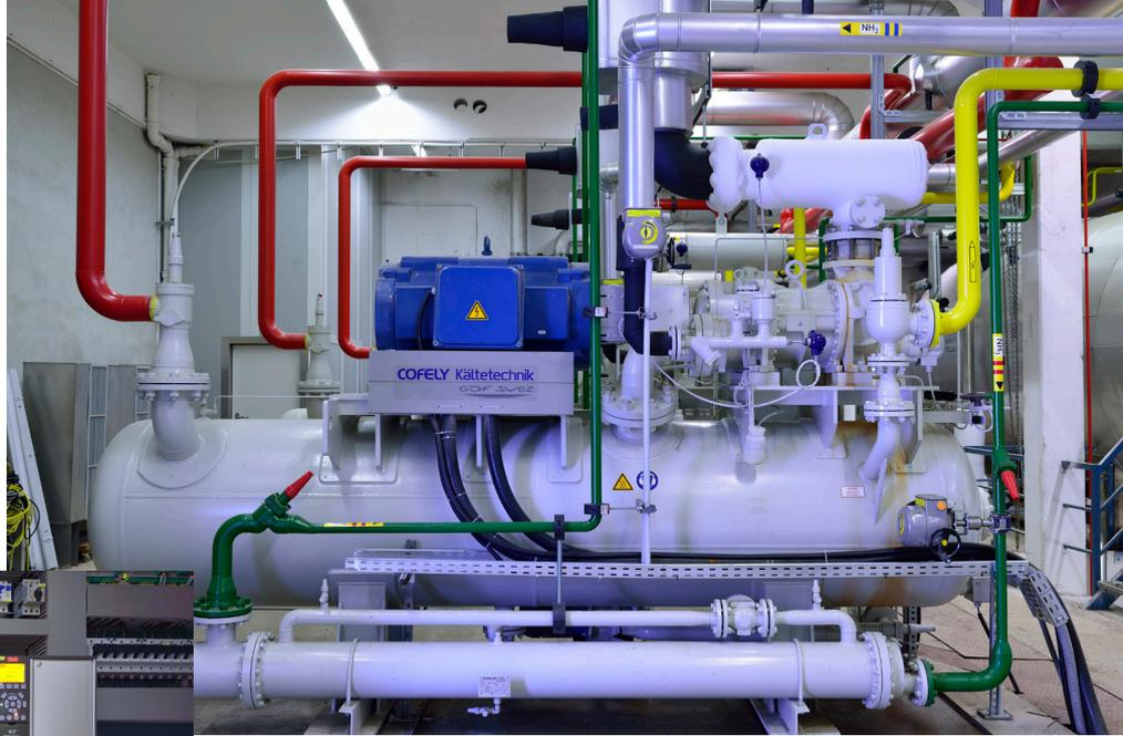
*Three screw compressors with a refrigerating capacity of 2,700 kW guarantee the required level of cooling, whereby a 315 kW Danfoss VLT® HVAC Drive frequency-controlled compressor drive supplies the base load.*
