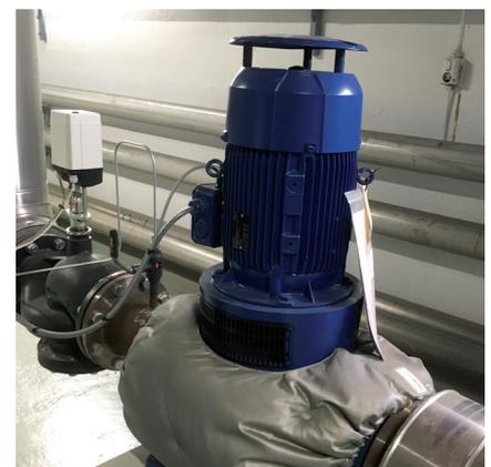
*The drive reduces the speed of the process water distribution pump, which in turn reduces heat loss. In addition the insulation reduces heat loss even further, resulting in a double energy saving.*
