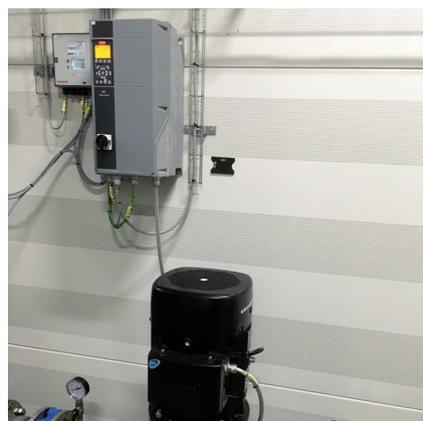
*VLT® AQUA Drive controls each pump for central heating water distribution, reducing energy consumption by up to 40% compared to direct-on-line operation. The process water pumps at a rate of 250-350 m<sup>3</sup>/h*
