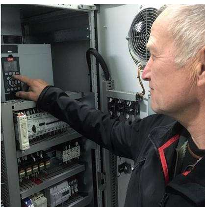
*A cabinet-mounted VLT® HVAC Drive controls each of the four powerful 500 kW heat pump compressors*
