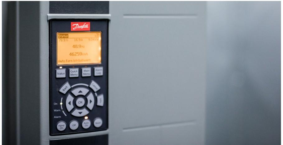
With frequency converters, the fans of the clinics' air-handling system can be operated up to 40 per cent more efficiently.
