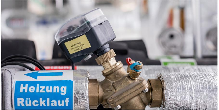
AB-QM balancing and regulating valve allows precise control of the water flow and reduces energy consumption.
