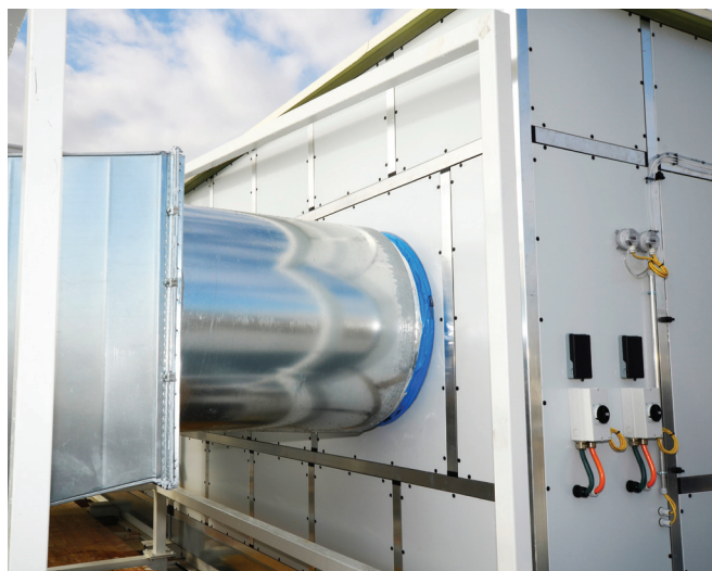
Connection between fan outlet and duct system
