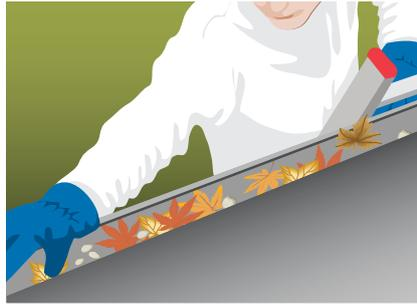
1. Ensure that the roof and the gutter system are heated and remove sharp edges, leaves and mud. Check and prepare the switchboard.
