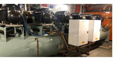
also mean there is no performance degradation over time, where oil-based chillers typically lose 10-30% of their capacity and efficiency over the life of the chiller, mainly caused by oil coating the heat exchangers and acting as an insulator which inhibits optimum heat transfer (see ASHRAE 601 paper for more details).
