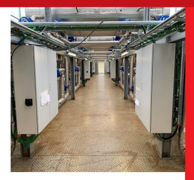
Two Turbocor<sup>®</sup>-powered Geoclima heat pumps HP02 and HP03 cool the flue gas to ensure the new scrubber's efficiency—and eliminate the need to provide the scrubber with an expensive external water supply. These heat pumps also cool the variable speed drives powering HP01 and the mechanical equipment room, recovering the heat from cooling these sources to the district heating system.
