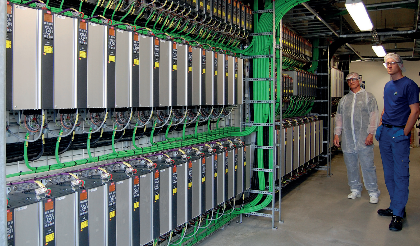
The 1400 VLT® drives are mounted in a series of well-ventilated control rooms, with no need for cabinets. From left Knud Rahbek and maintenance manager Simon Arentoft
