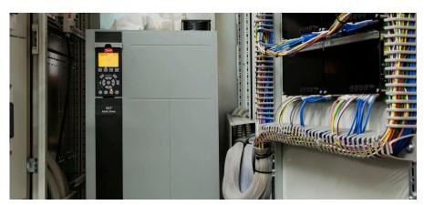
Danfoss Drives VLT® FC102 250 kW drive mounted inside its cubicle.
