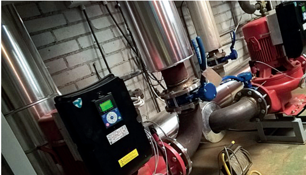
VACON® 20 Cold Plate integrated with Kolmeks' updated family of in-line pumps with 7.5 kW (3-phase) motor.
