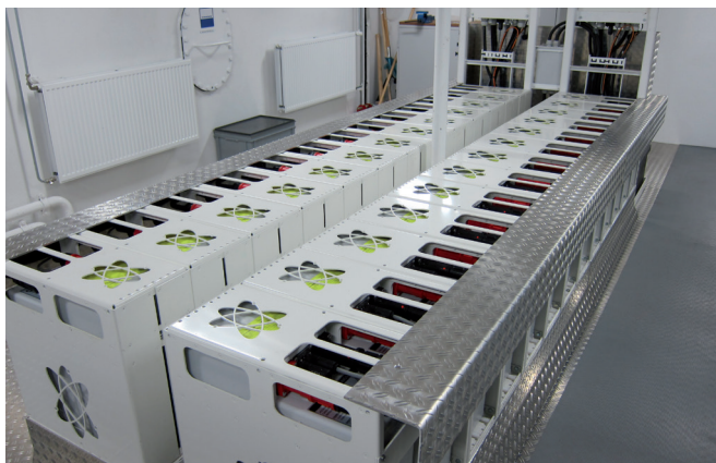
The 2 x 68 kWh Li-Ion EST-Floattech Battery system with battery management system.
