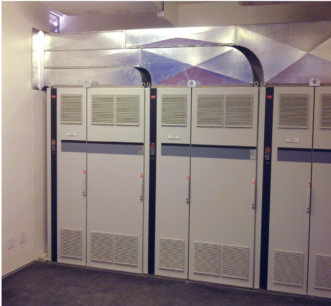
These VLT® AutomationDrive frequency converters with back channel cooling control motors in the mine dewatering system. They are installed in the MCC substation.
