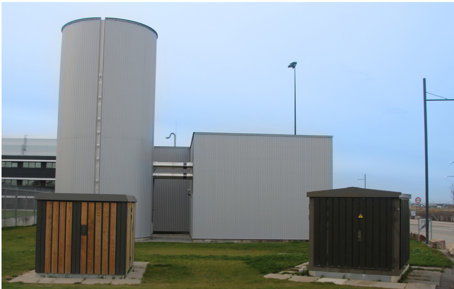
The FlexHeat plant stores thermal energy corresponding to a virtual battery of 4 MWh in the 100-m 3 storage tank on the left side of the image.
