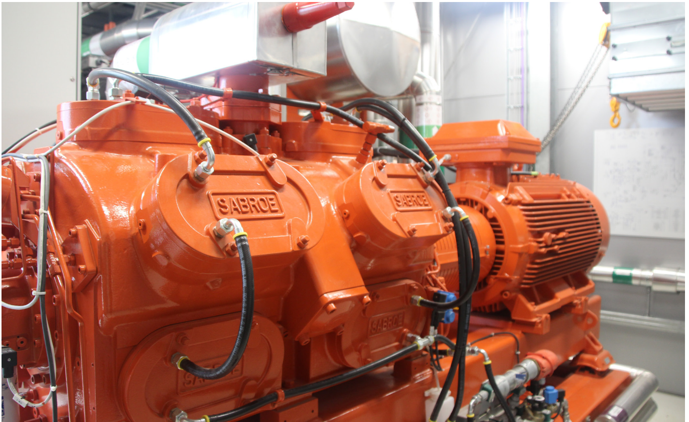
The variable speed drive-controlled heat pump sends 70°C – 80°C water out into the system, and approximately 40 °C water comes back to the plant. The plant was supplied and installed by Johnson Controls Aps with consultancy from COWI A/S.
