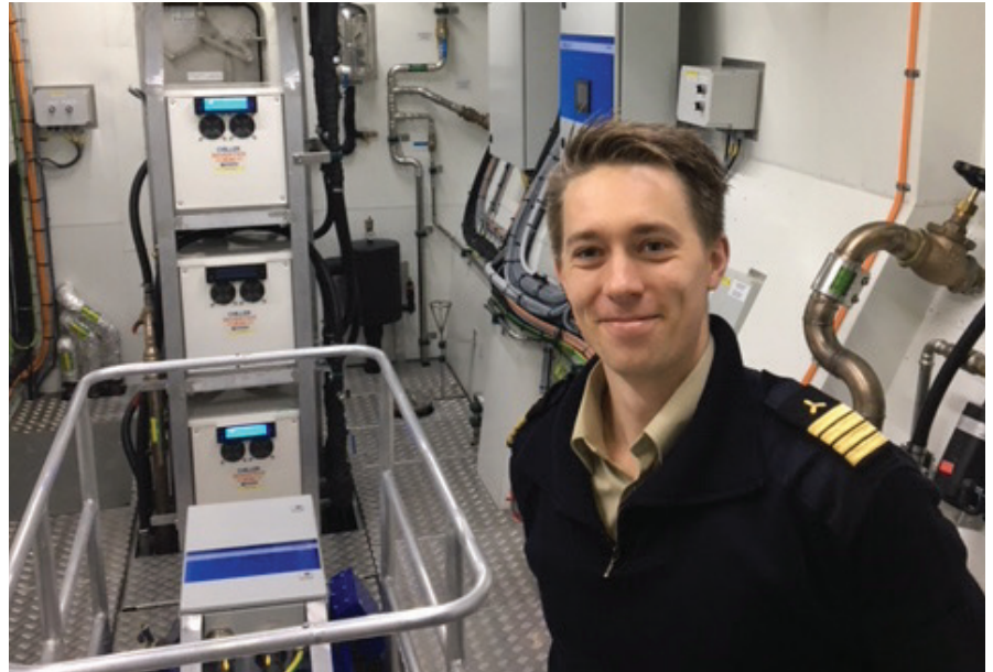
Lars Haugnes is highly satisfied with the performance of Danfoss drives and instrumentation installed in the machine room of Future of the Fjords , contributing significantly to protecting the pristine fjord environment.
