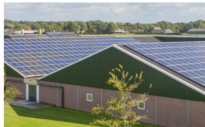
▲ Roof-mounted solar panels
