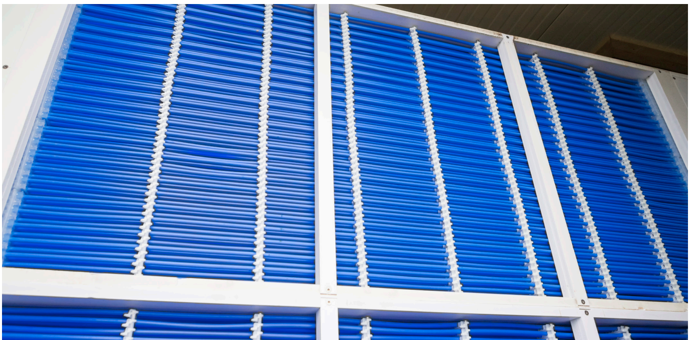
▲ Exegy corrosion-free heat exchangers installed by Inno+ as part of the advanced climate and heat recovery system.
