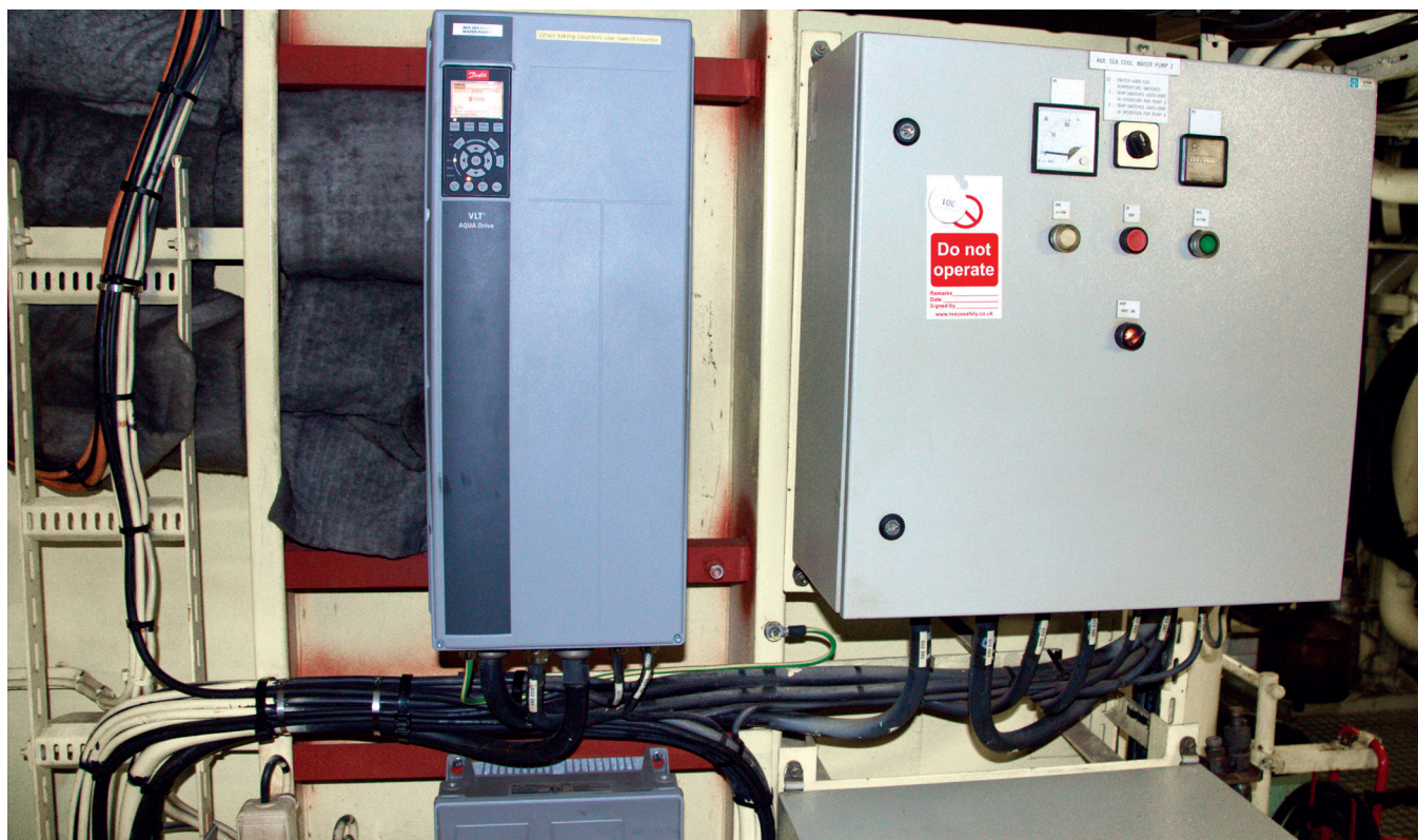
The sea water cooling pumps and engine room ventilation systems onboard the vessel are powered by Danfoss drives.
