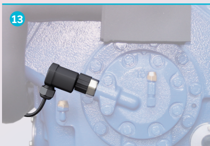
Oil differential pressure sensor
