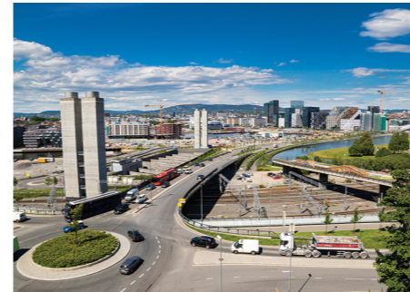
Bjørvika tunnel Oslo, Norway
